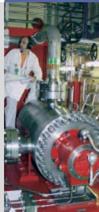
Security calls for inspections (Photo Axpo)
